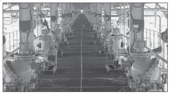
The next photograph shows a typical gantry position. From left to right, there is a supply line attached to an isolation valve, a second isolation valve and piping leading vertically to the loading arm. The meter is equipped with a dual channel, quadrature pulse
