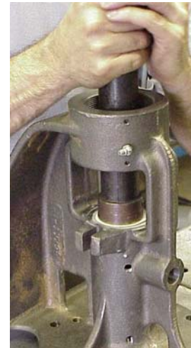
Figure 8, Installing the inner seal seat retainer
